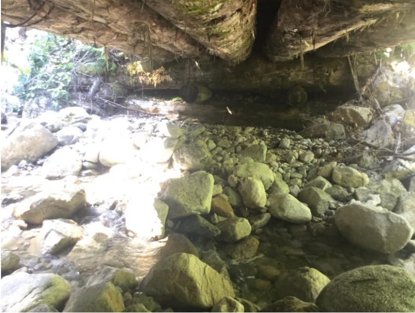
Left Bank Abutment
