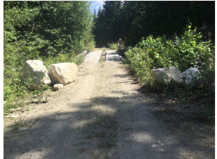
Left Approach Facing Bridge
