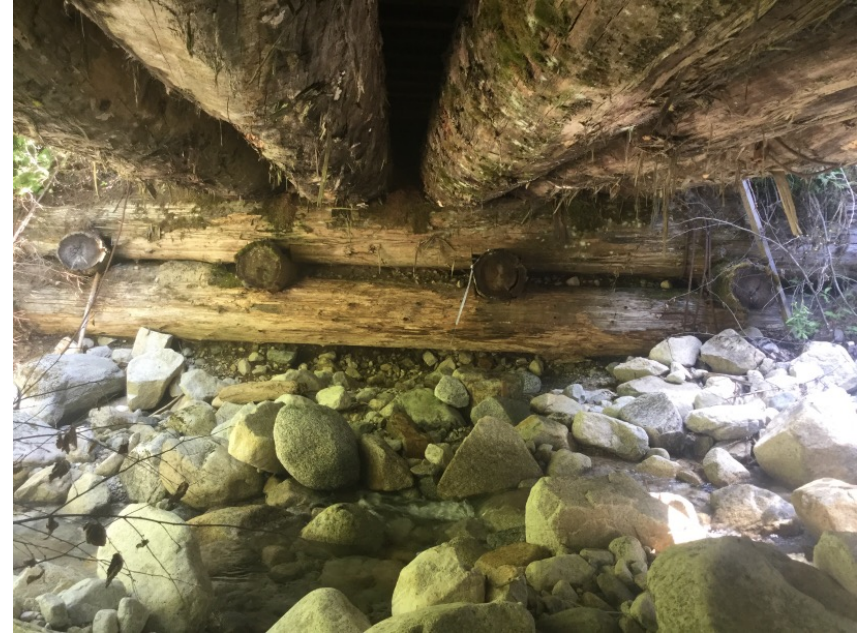
Right Bank Abutment
