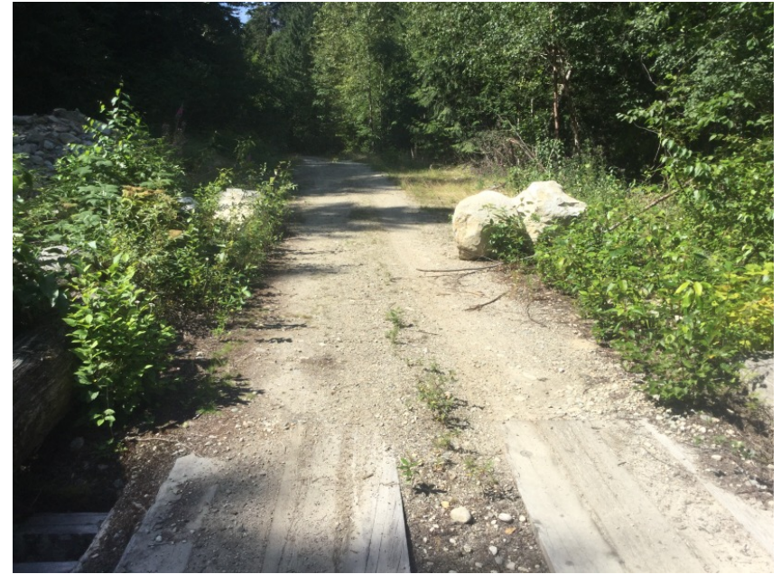
Left Approach Facing Away From Bridge
