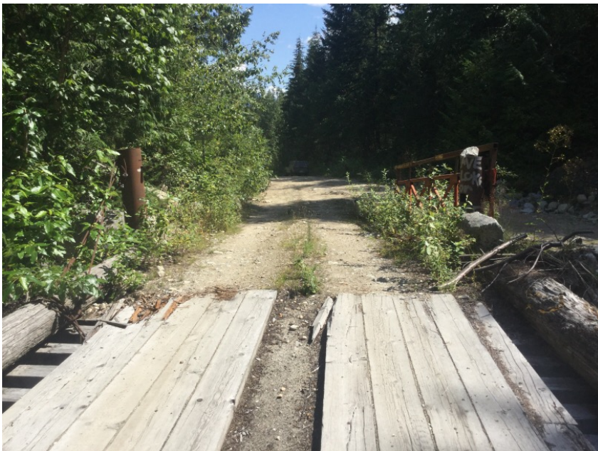
Right Approach Facing Away From Bridge
